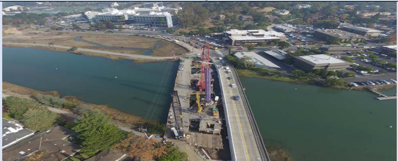
Aerial View of Pier CIDH Piling Foundation Construction
