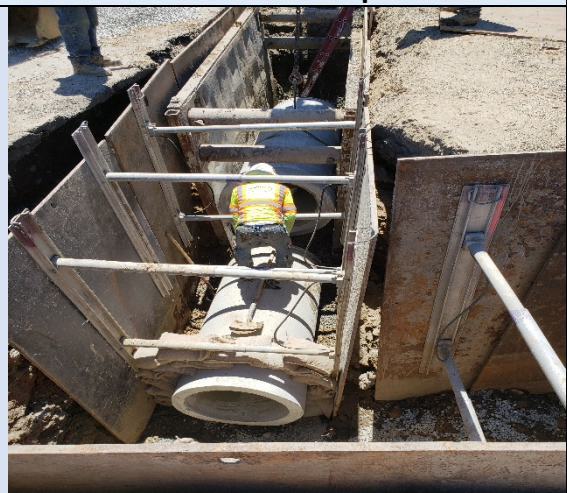
30-inch RCP Storm Drain Pipe Installation
