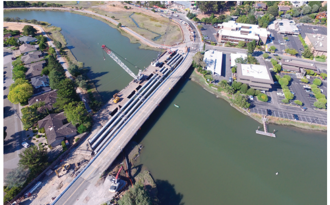
Stage 1 girder installation.
